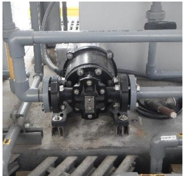
Figure 4 –Eclipse series E25 and E125 Hypo Pumps metering Sodium Hypochlorite (NaOCl) provide pulseless, laminar flow with smaller piping and without the need for dampeners
